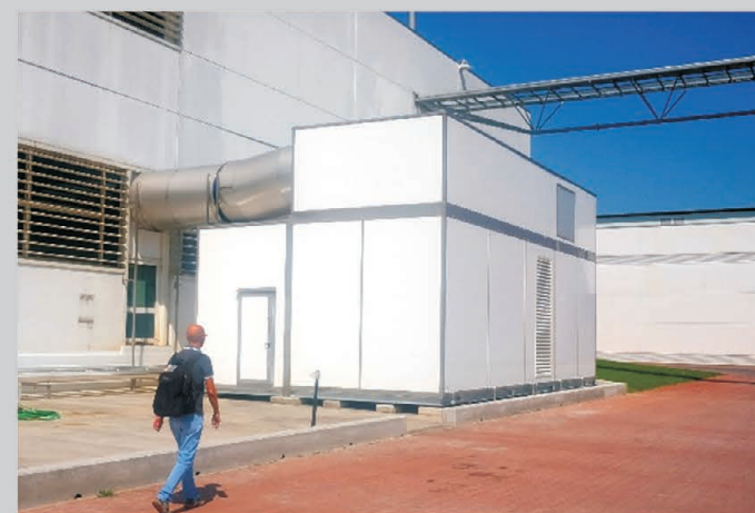
HIGH CAPACITY AHU WITH VESTIBULE AND INTEGRATED DUCTS
